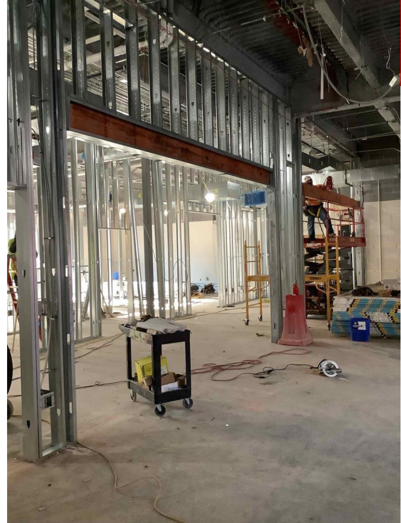
Cafeteria wall framing and wood blocking
