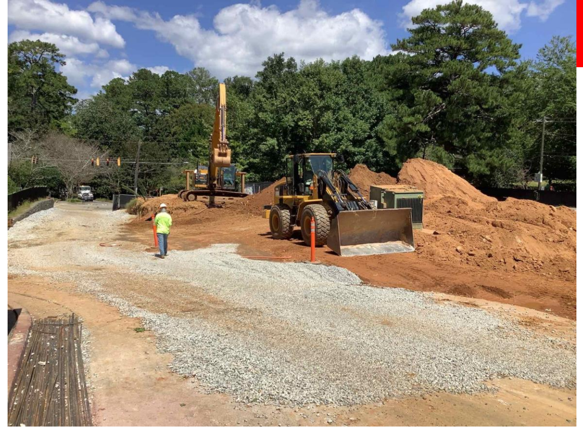
Building pad grading
